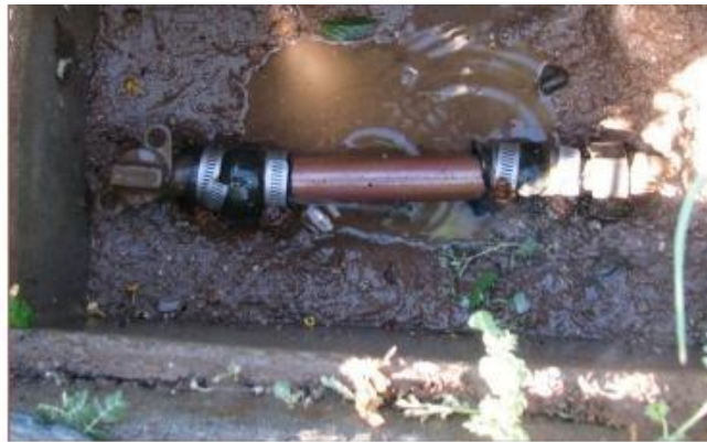
Water meter removed and replaced with straight pipe.
