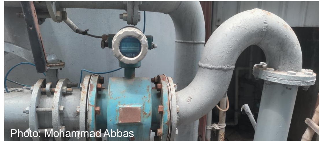
Swirl caused by two bends in different planes
