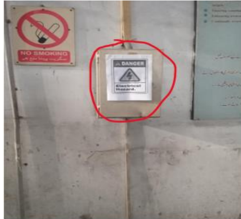
Fixing of safety symbols on DB boards
