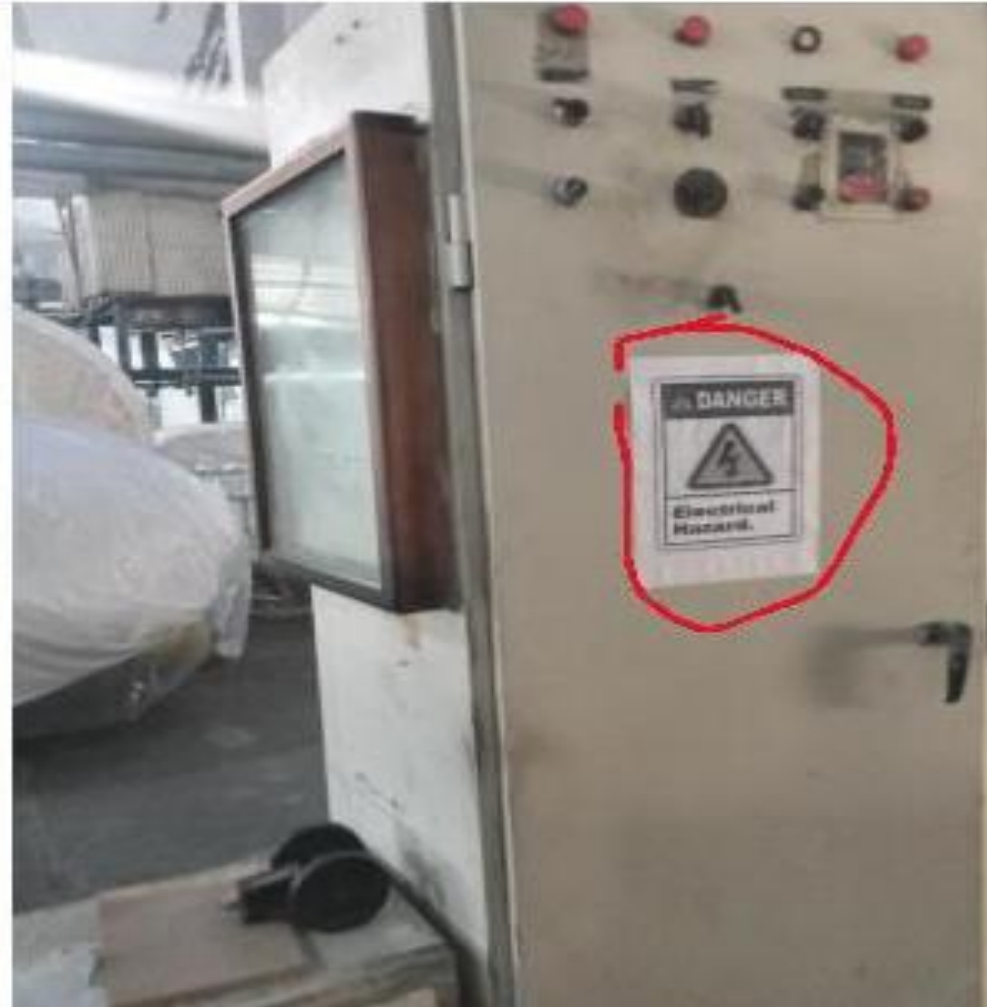
Fixing of safety symbols on DB boards
