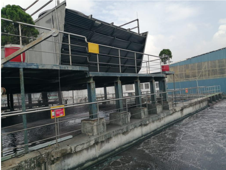
Cooling tower at aeration tank inlet
