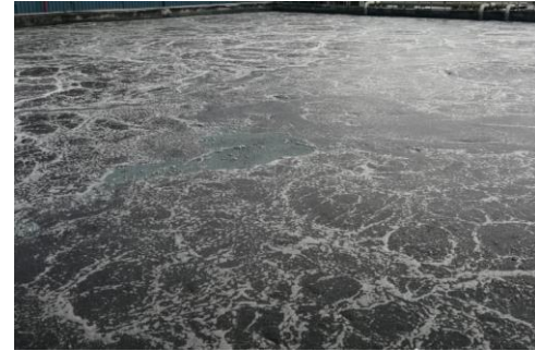
Fine bubble aeration with only gentle agitation at top
