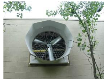
General ventilation of workfloor
