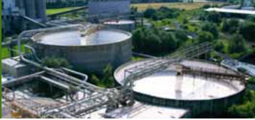
Slurry storage tanks
