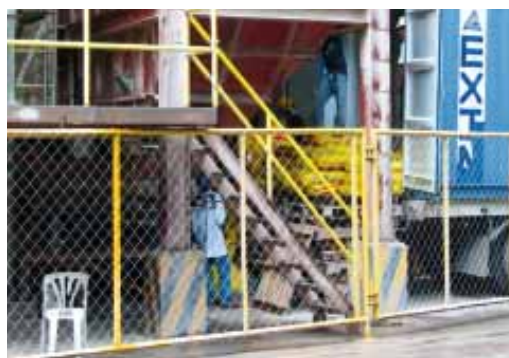
The semi-automatic co-processing facility for solid waste
