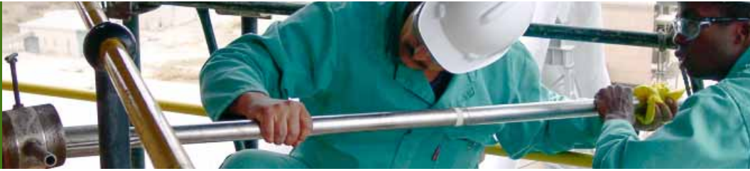
A measuring team working on a main stack in South Africa
