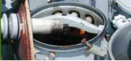
Future co-processing potential: PBCs from transformers
