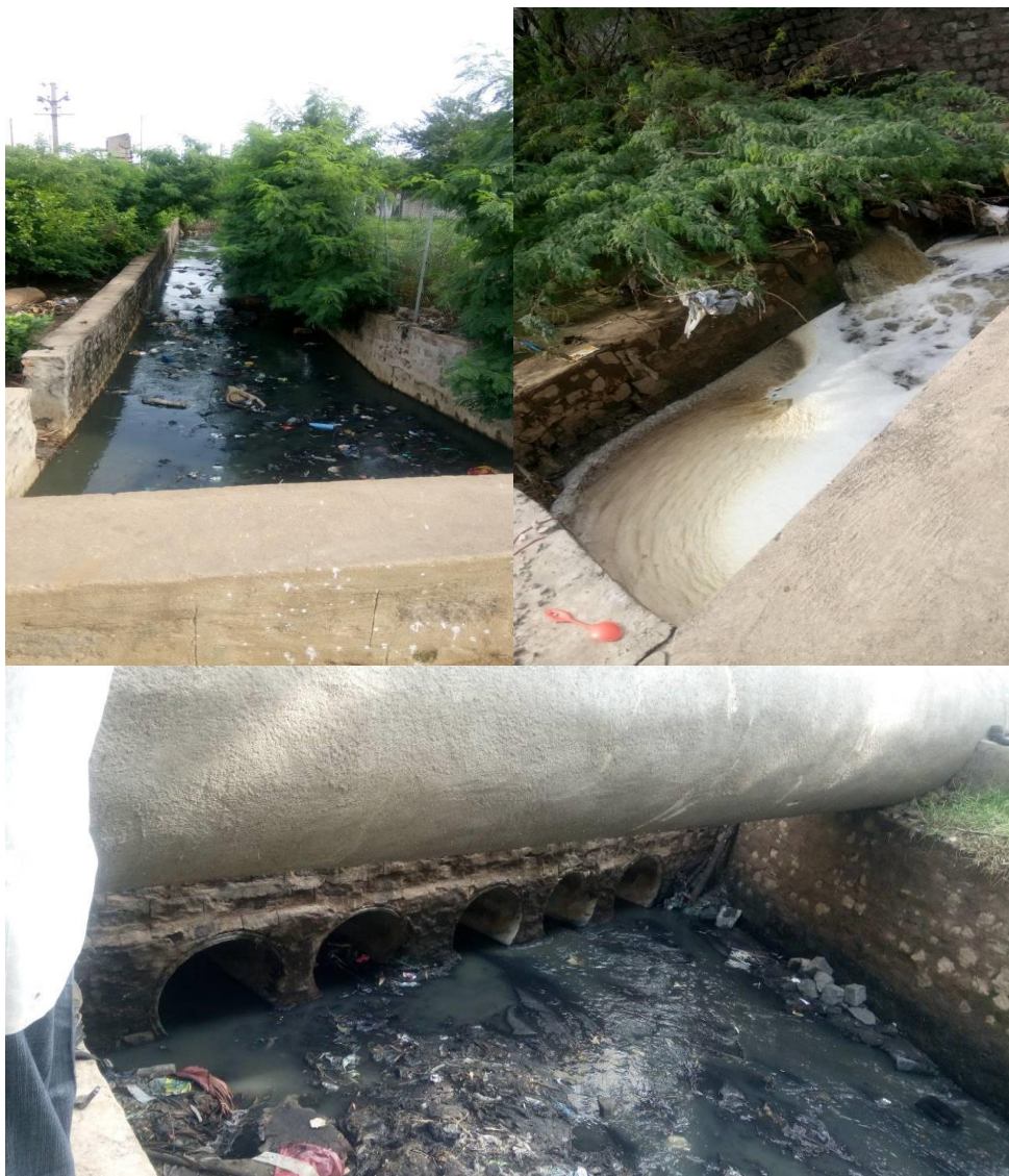
FIGURE 7: SEWER DRAINS IN IP JEEDIMETLA, WHICH OVERFLOWS DURING HEAVY RAINFALL FURTHER POLLUTING THE NEARBY AREAS
