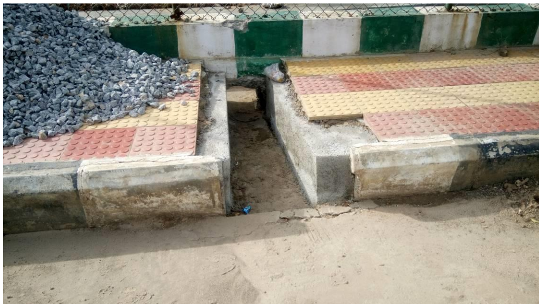
FIGURE 14: STRUCTURES CONSTRUCTED TO DIVERT WATER FROM ROAD TO THE DRAINS
