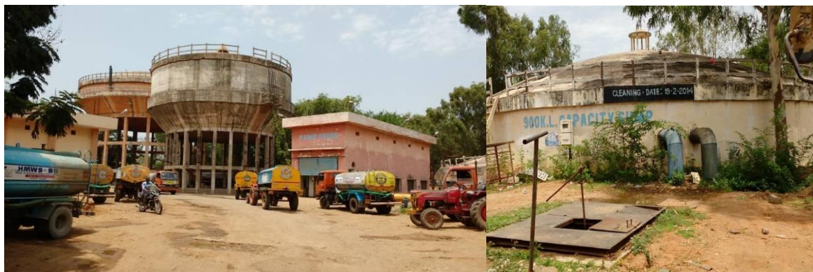
FIGURE 15: WATER TANKS IN IP JEEDIMETLA
